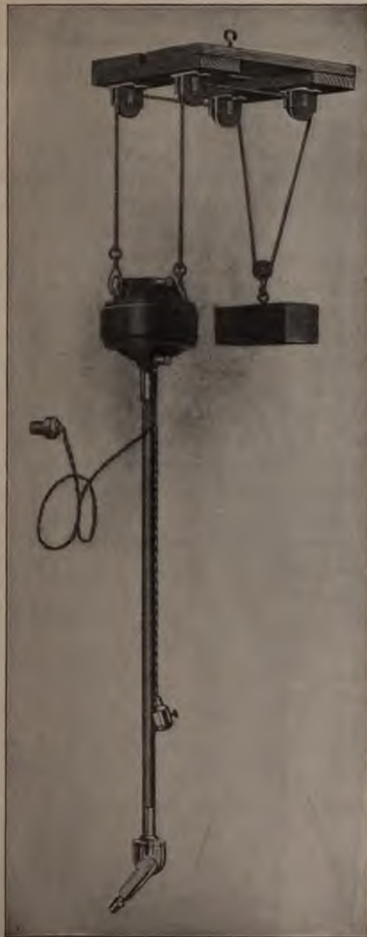
FIG. 51.—Electric concussion-hammer.
